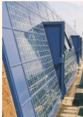
The Photovoltaic roof on the University of Reading's engineering department building.
