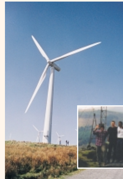
A modern wind farm
